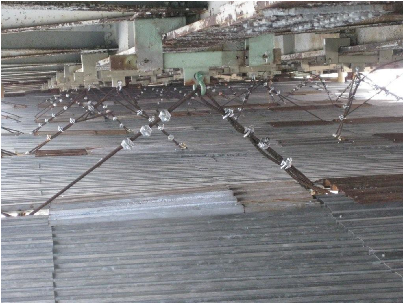
Cable/Metal Deck Platform Below Roadway, Tie Ups & Beam Flange Clamp Hangers
