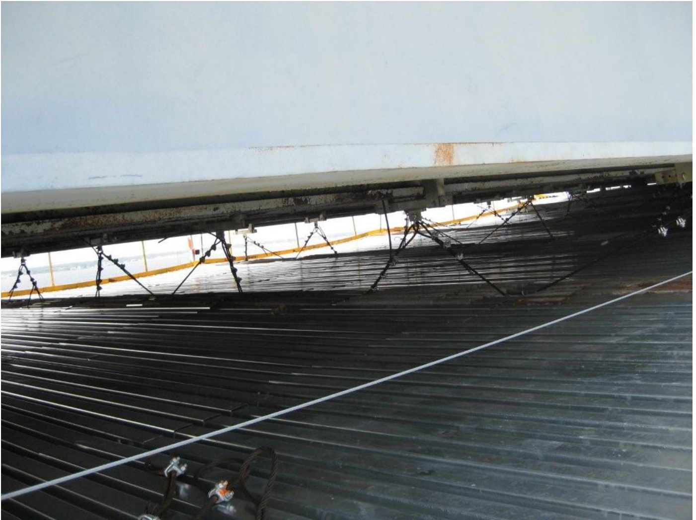
Cable/Metal Deck Platform Below Roadway
