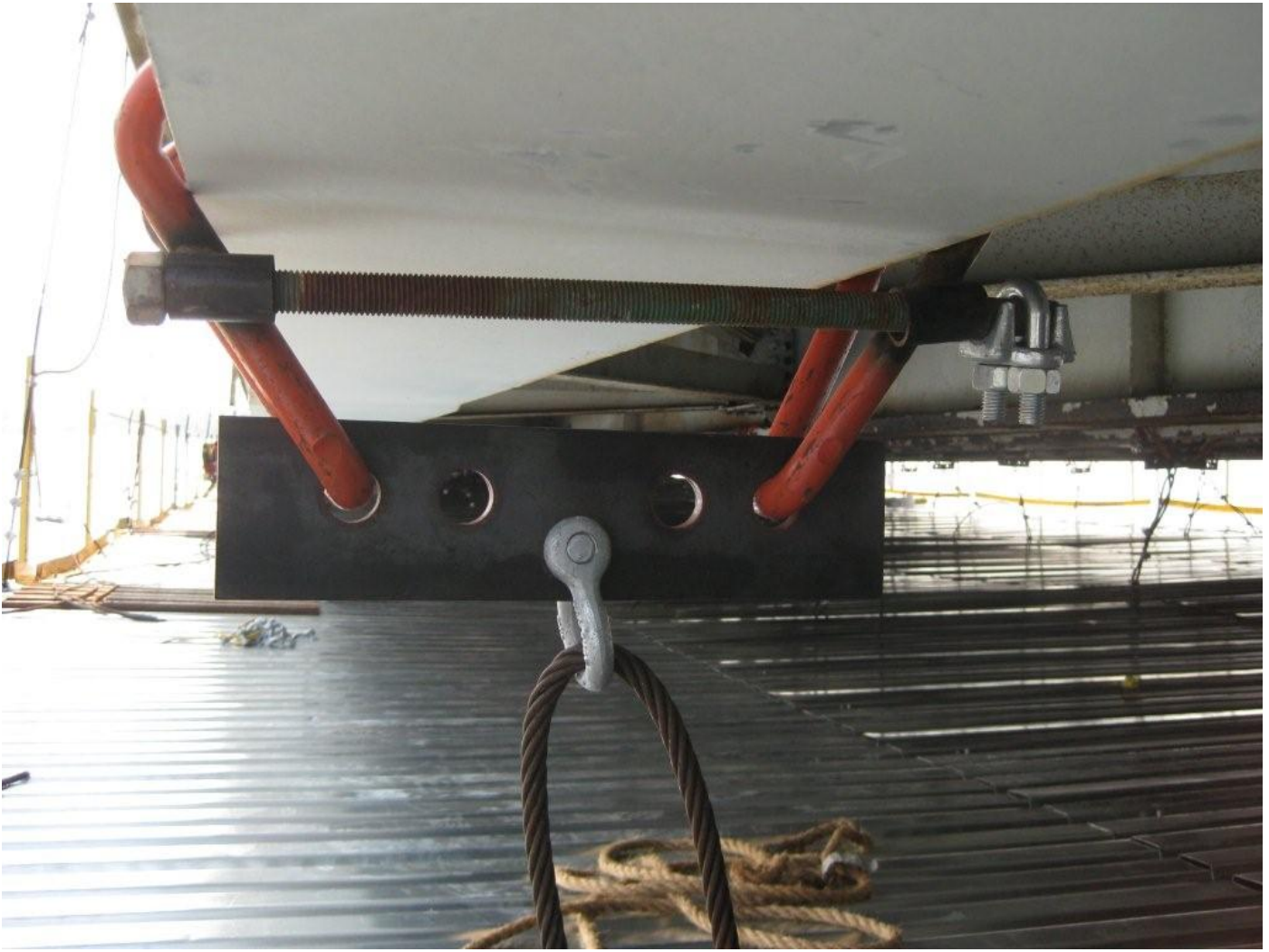
Cable/Metal Deck Platform Below Roadway & Beam Flange Clamp Hanger Assembly
