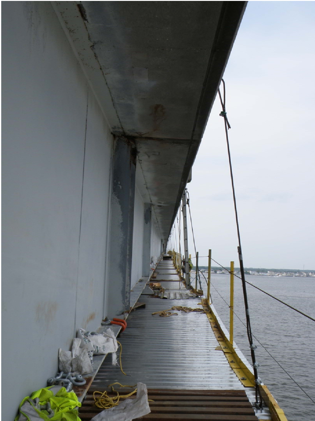
Cable/Metal Deck Platform Below Roadway
