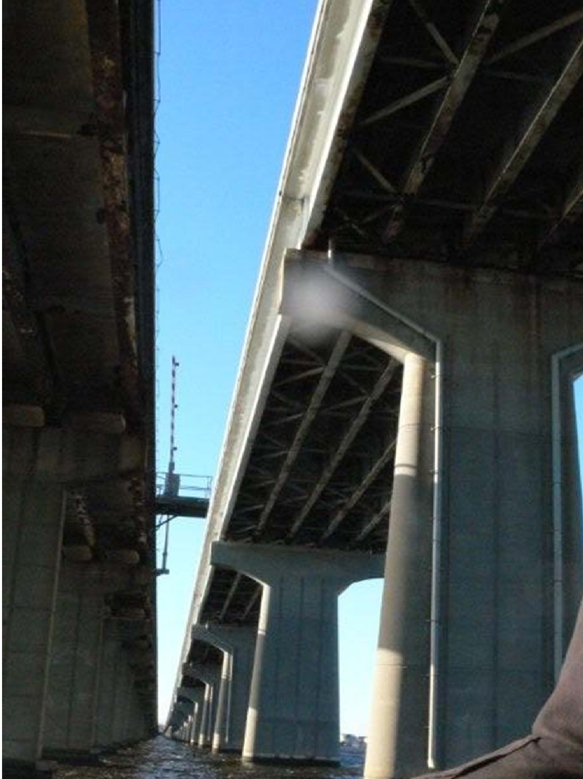
Steel Girder Bridge
