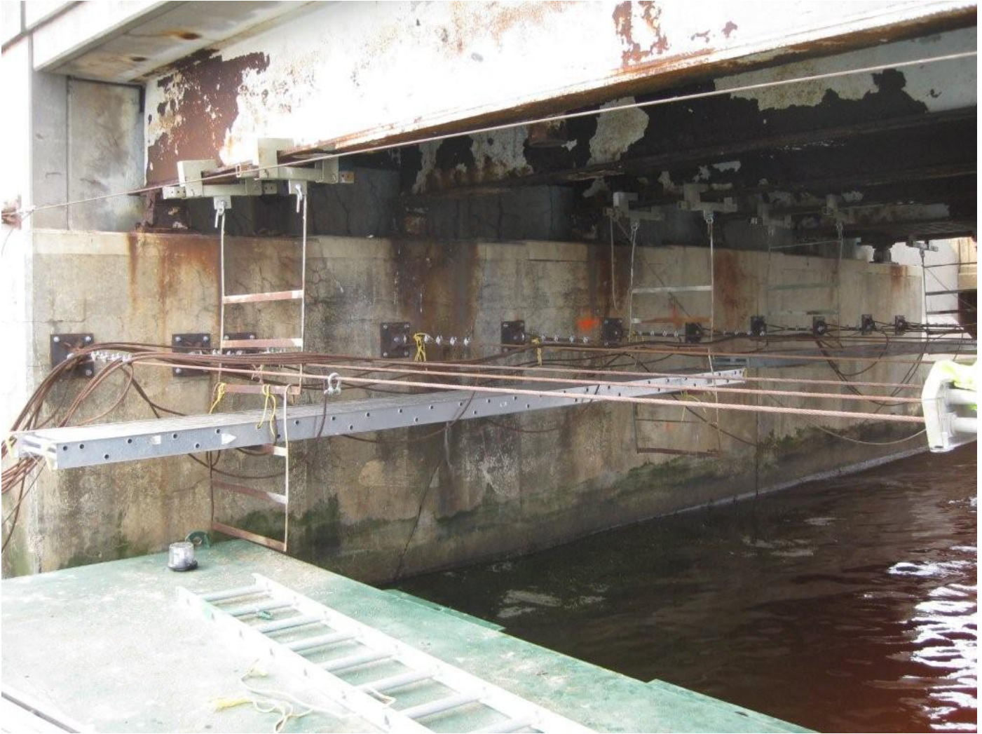
Anchor Plate End Support Assemblies Main Cables
