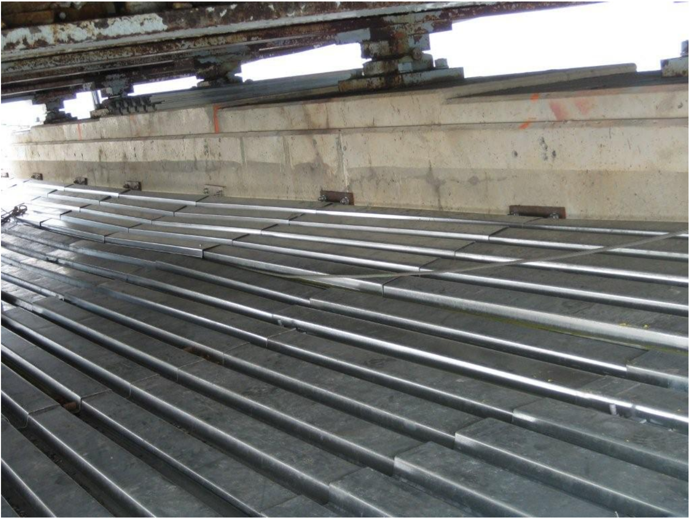
Cable/Metal Deck Platform Below Roadway & Anchor Plate Assemblies
