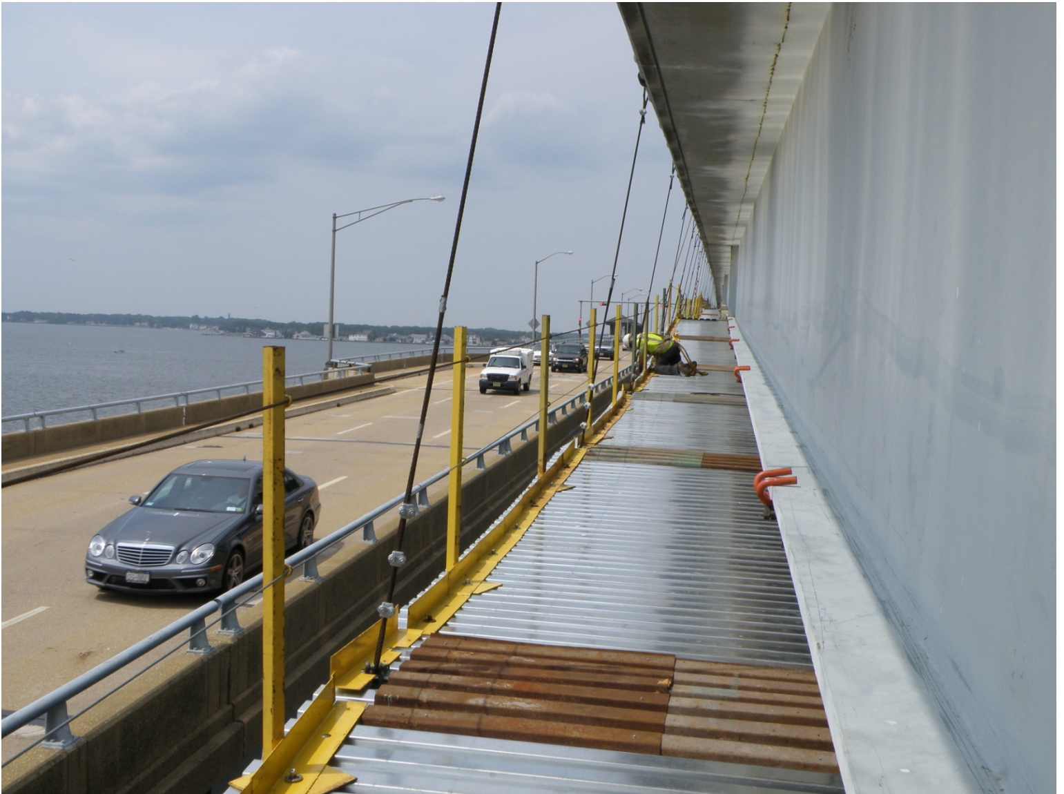
Cable/Metal Deck Platform Below Roadway
