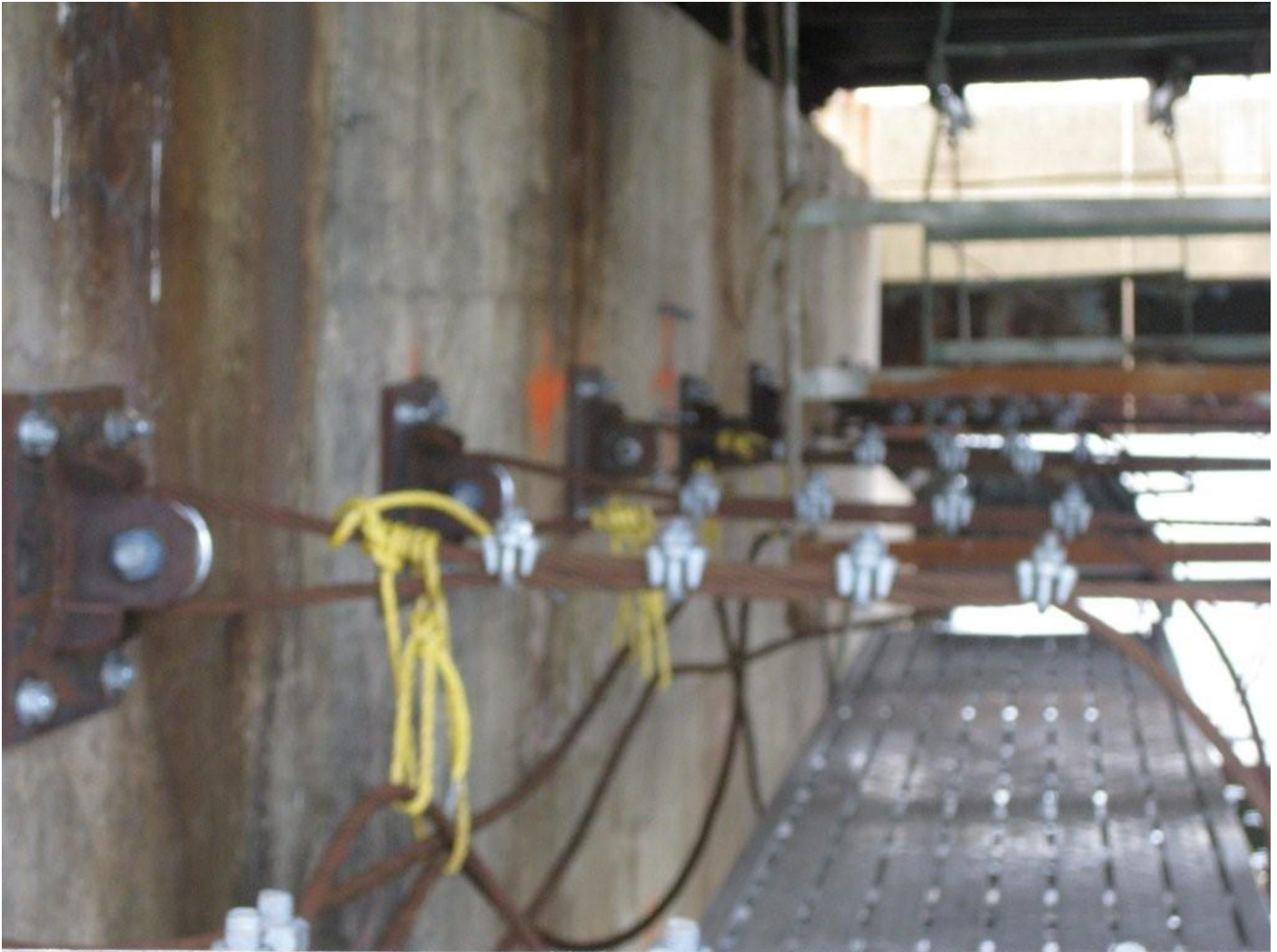
Anchor Plate End Support Assemblies Main Cables
